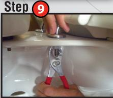
Secure the seat using pliers...
